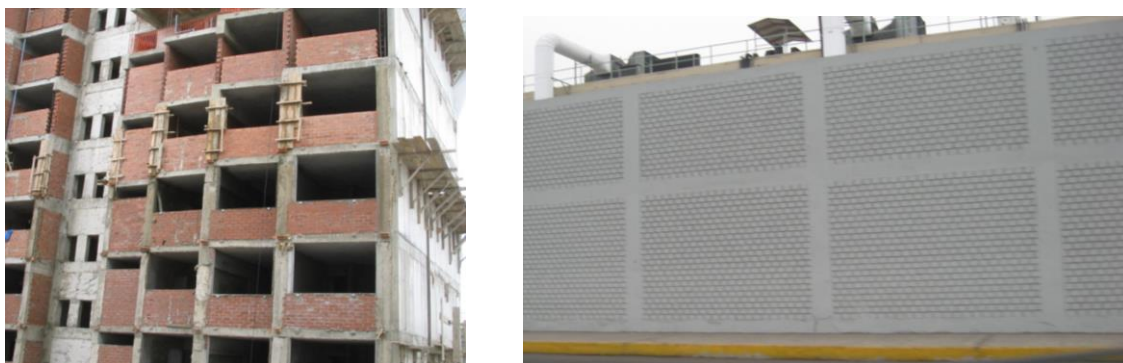
Fig. 9 – Non-structural masonry walls: parapets and fences.
