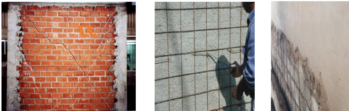
Fig. 5 – Confined masonry wall tested and repaired with wire meshes [11].
