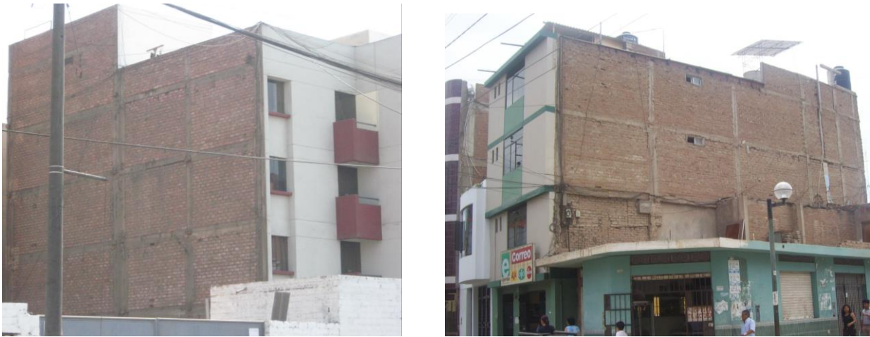
Fig. 2 – Popular multistory housing buildings with confined masonry walls.
