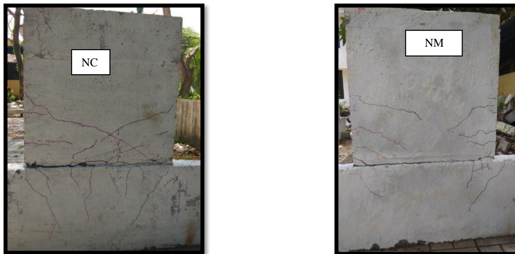
Fig. 9 –Crack Pattern for specimen NC and NM
