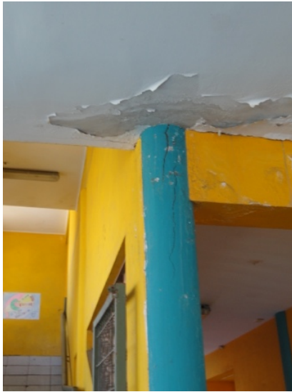
(a) Cracking originated by rotation of the wall-beam connection
