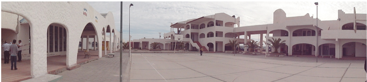
Figure 5. General view of the complex Marítima School, Tongoy
