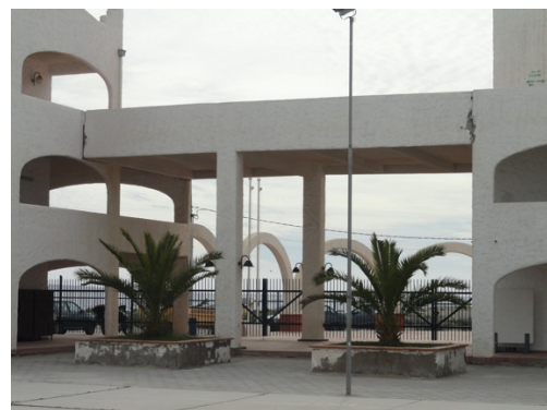
(b) Damage in the bridge connection
