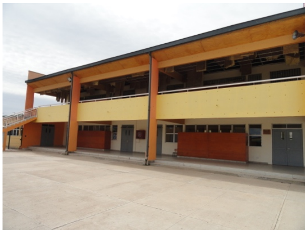
(a) General view of the west wing
