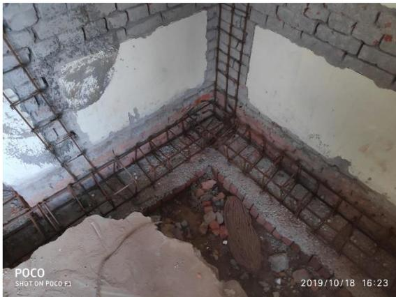
(a) Excavation of the plinth beam for Splint
