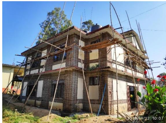
(b) Fixing of reinforced bar mesh Splint and bandage on outer walls of the building
