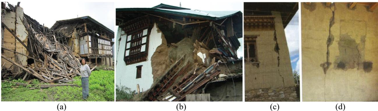
Fig. 1 – Rammed earth buildings damaged by 2011 earthquake: (a) Out-of-plane wall collapse; (b) Corner overturning; (c) Corner crack; (d) Vertical crack under loading point of floor joist.
