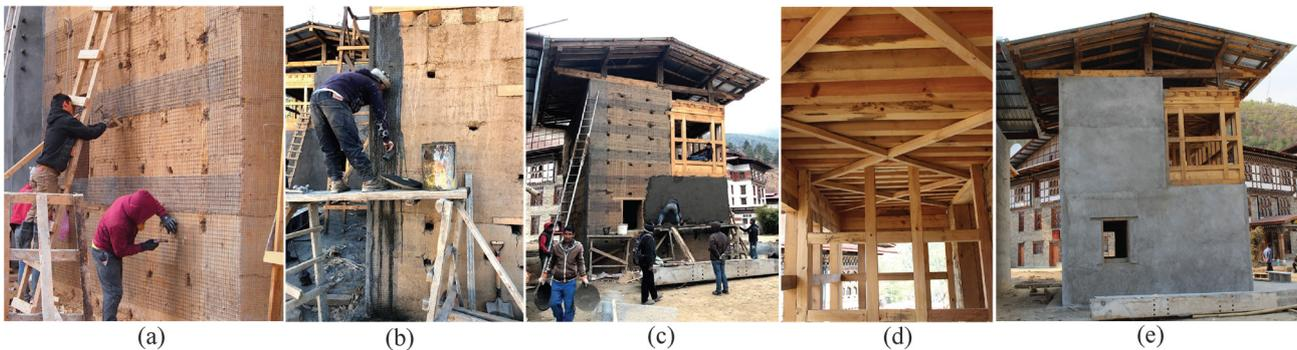
Fig. 5 – Retrofitting work details: (a) Fixing mesh; (b) Wetting wall surface with cement slurry; (c) Applying cement plaster; (d) Providing bracing under floor joists; (e) Final view of building after retrofitting work.
