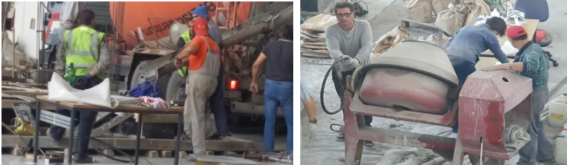
Fig. 1 - Photos taken during concreting of models.
