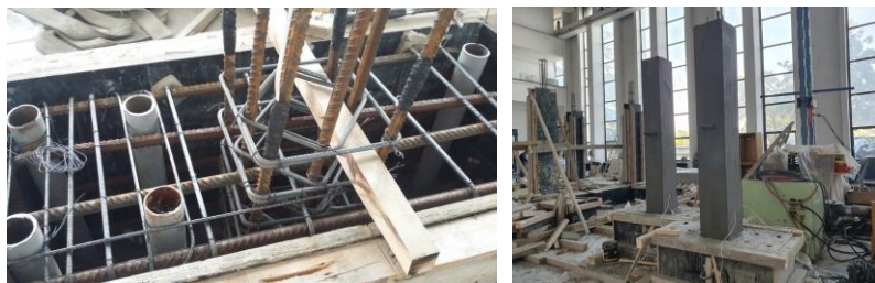
Fig. 6 - Construction of the column models (Model M1 and Model M2) for experimental tests.
