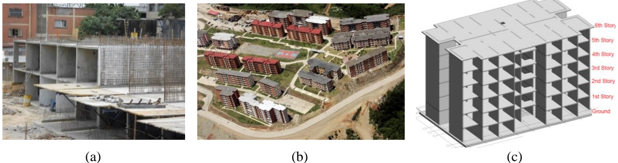
Fig. 1 - (a) Tunnel construction in Caracas; (b) Case-study building in Ciudad Caribia Development (6 Ha), conceived to have 37 residential buildings (660 family units) [3]; and (c) Case-study building isometric.
