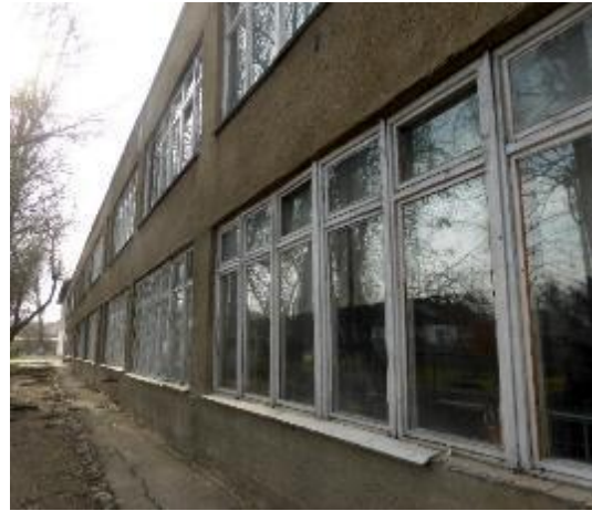
Fig. 3 – Typical precast RC school building in the KR (Type 5): a) precast RC beams, columns, and the connections, and b) exterior view of the building showing precast RC panels [1]
