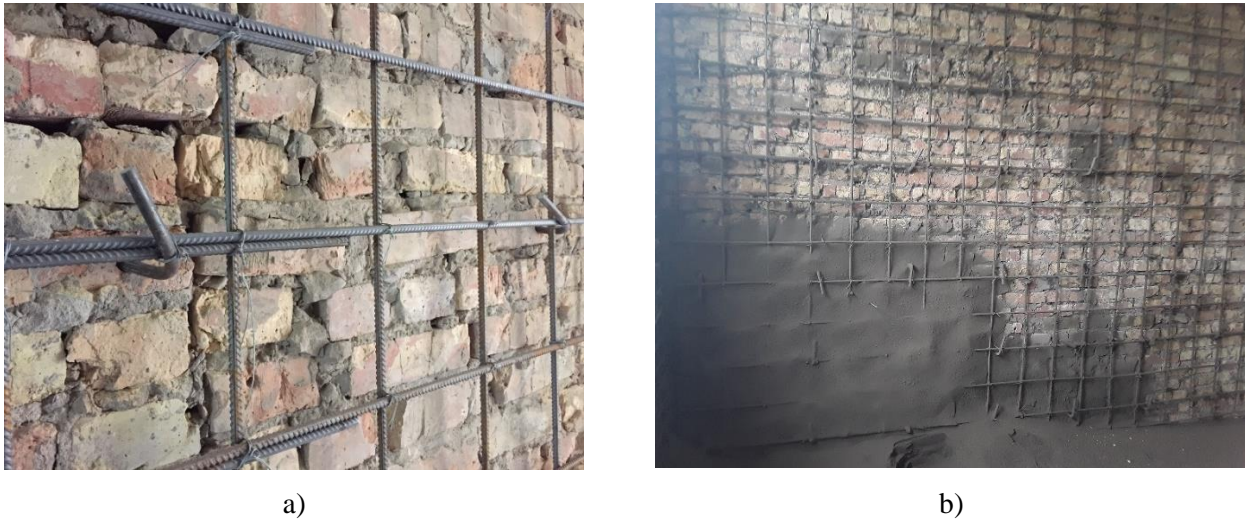
Fig. 7 – Features of RC jacketing technique: a) wall reinforcement and anchors, and b) shotcrete application (photos: S. Brzev and U. Begaliev) [1]
