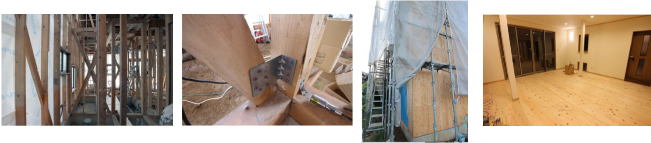
Fig. 2 – photo images during the construction work: columns at 1F on Aug. 5 th (left), a joint at 1F on Aug. 7 th (left middle), outer wall on Aug. 11st 11 (right middle), and a room at 1F on Oct. 25 th (right)
