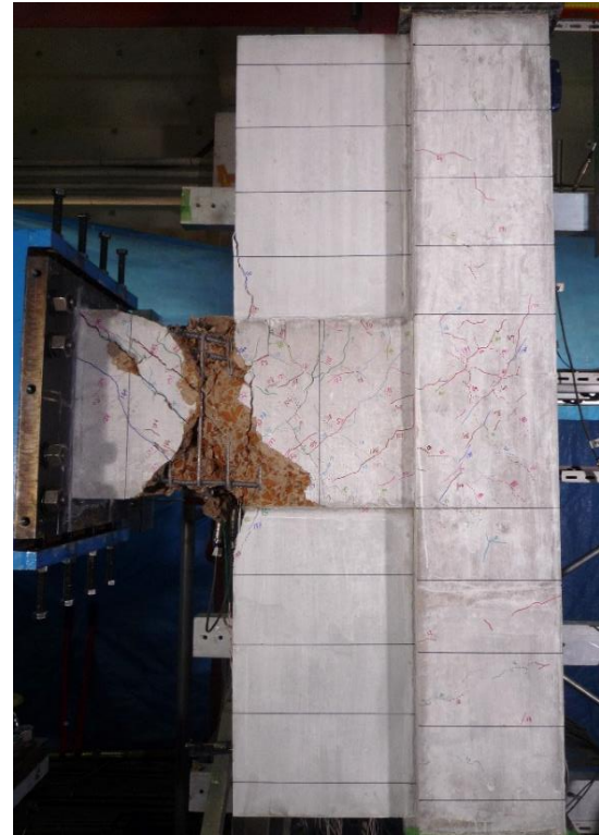
Fig. 5 – Damage to the specimen J1-W
