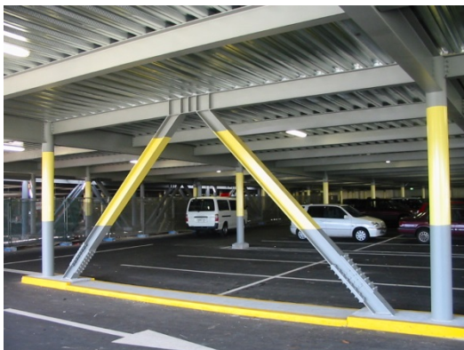
(a) EBF with continuous active link and (b) EBF with bolted replaceable active link collector beam
