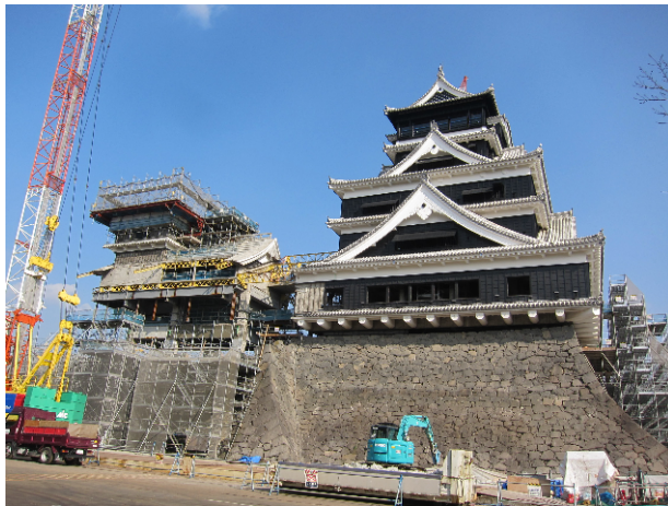
Fig.3 – Restoration Construction Site
