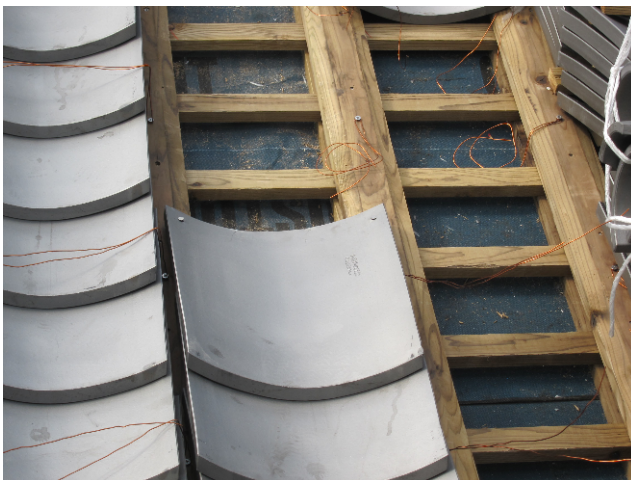
Fig.16 – Connection of plain type roof tiles
