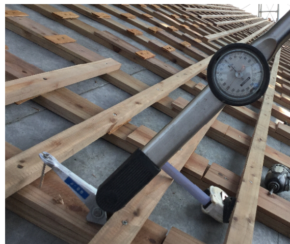
Fig.17 – Inspection of nail Strength
