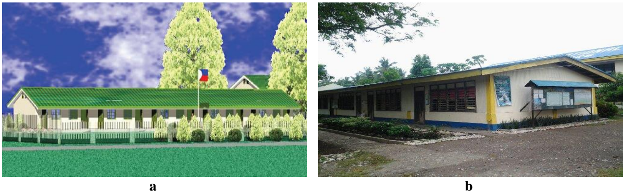
Figure 4 – Single storey reinforced concrete, 5-classroom index buildings with various seismic design provisions a) RC2/LR(1)/MD, b) RC2/LR(1)/LD
