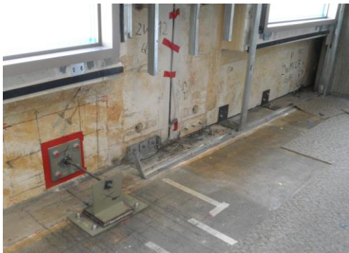
Fig. 12 Modified cladding panel bottom connection
