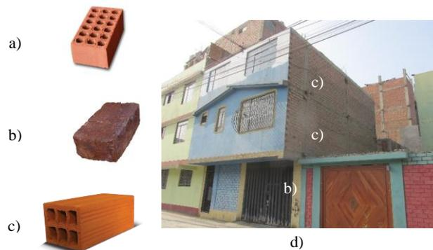
Fig. 1 – Types of bricks used in non-engineered confined masonry dwellings: a) hollow, b) solid c) tubular bricks d) Solid bricks used in first floor and tubular bricks in upper floors.
