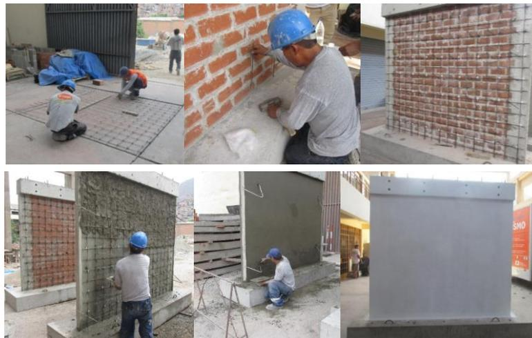
Fig. 2 – Retrofitting of confined masonry walls
