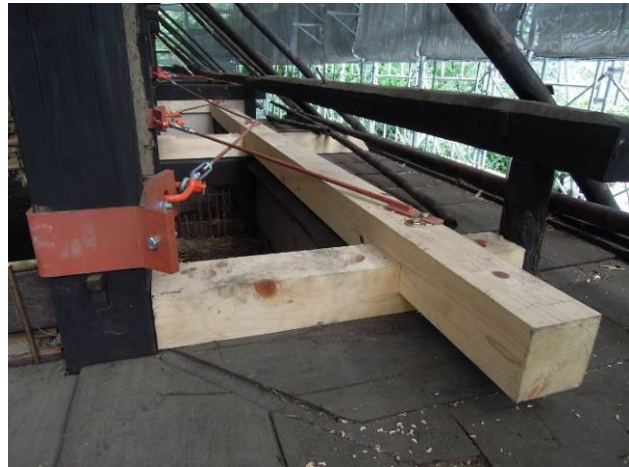
Fig.18- Floorboards nailed obliquely, Fig.19- Steel bar brace for horizontal plane
