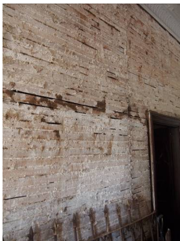
Fig.5-Plaster wall that is peeled off, Fig.6-Earthen wall that is peeled off
