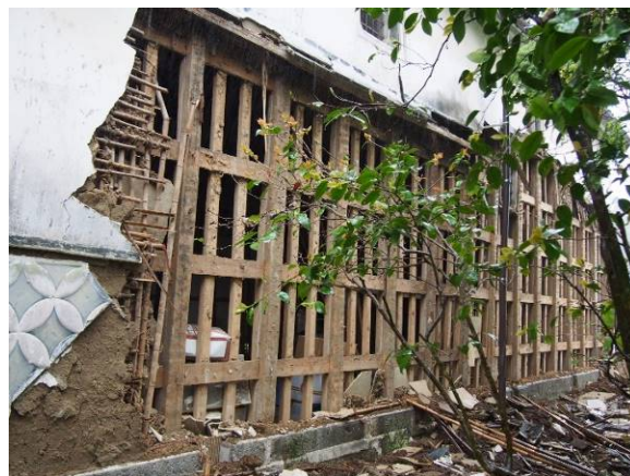
Fig.5-Plaster wall that is peeled off, Fig.6-Earthen wall that is peeled off
