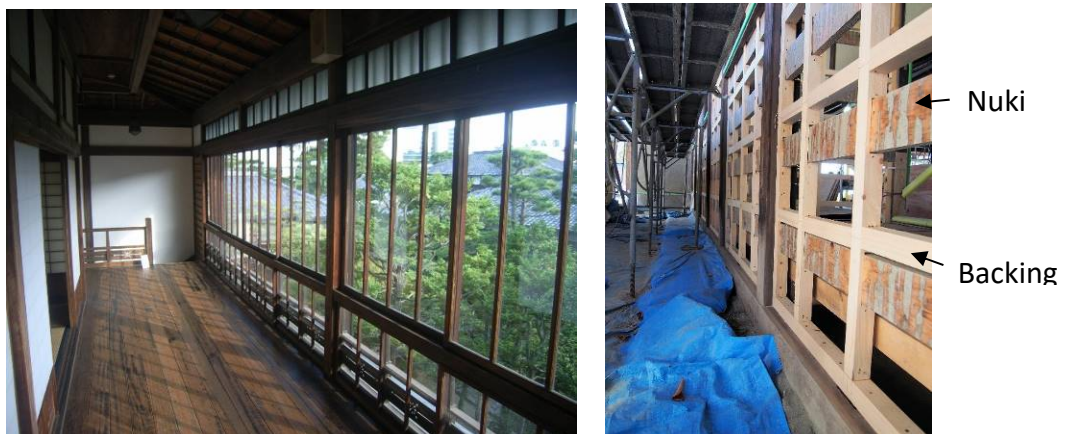
Fig.2-Openness of Japanese historical wooden buildings, Fig.3-Installation of backing material
