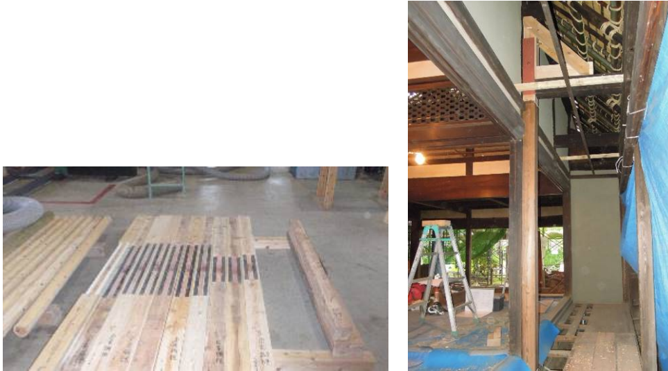
Fig.11- Specimens of reinforced columns, Fig.12-Attached additional pillar
