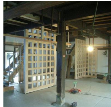
Fig.4-1- Degrading of maximum shear strength, Fig.4-2-Example of lattice wall
