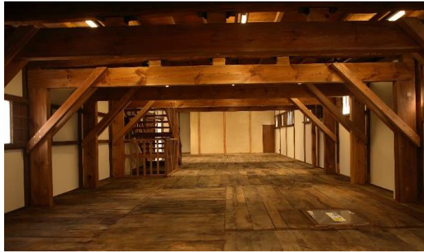
Fig.7-Rigid frame that is consisted of knee brace
