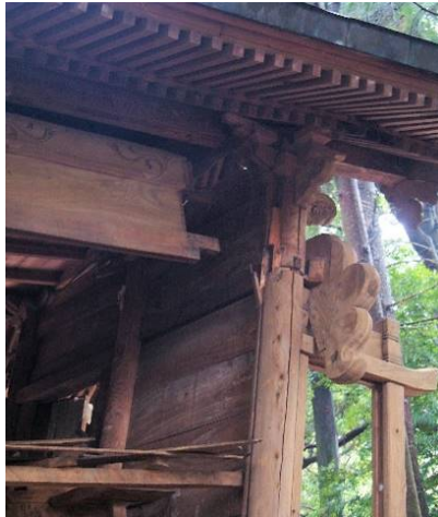
Fig.14-Disengagement of connections, Fig.15- Pin and wedge of connections
