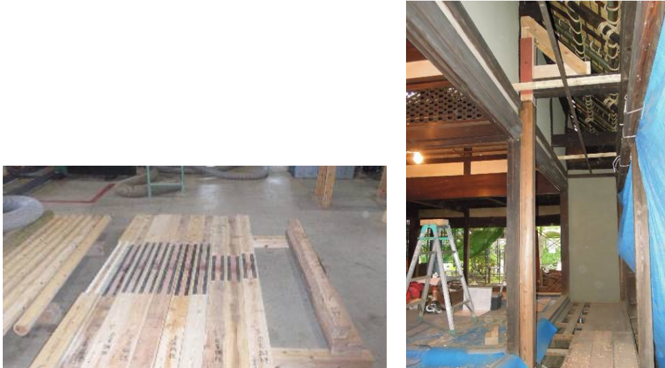
Fig.11- Specimens of reinforced columns, Fig.12-Attached additional pillar
