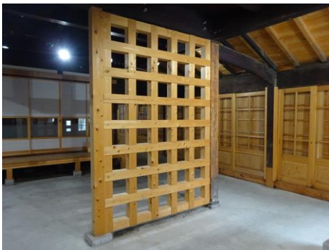
Fig. 12 – Installation example of the timber grid wall
