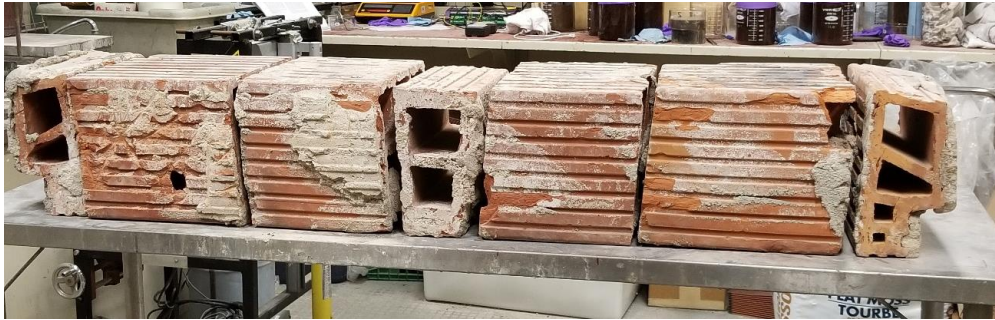
Fig. 6 – Extracted terracotta tiles from the Centre Block
