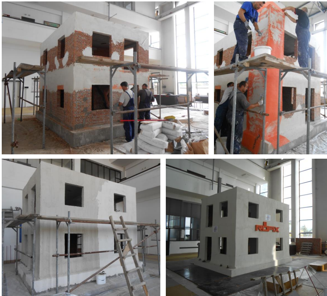
Fig. 5 – Retrofitting of the model using System RÖFIX SismaCalce
