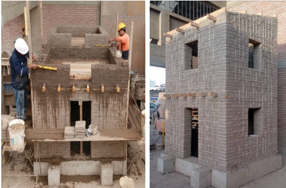
Fig. 4 – Construction of a half-scale reinforced adobe model.
