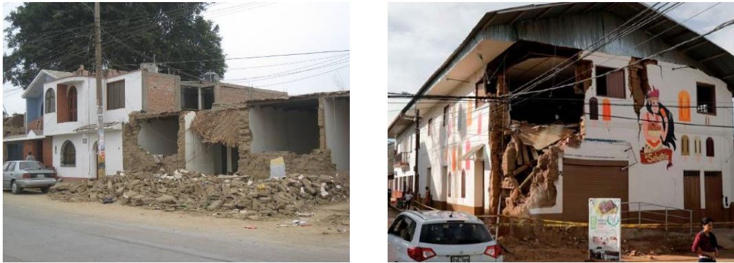
Fig. 1 – Adobe buildings heavily damaged by the Pisco, 2007 earthquake in Peru.
