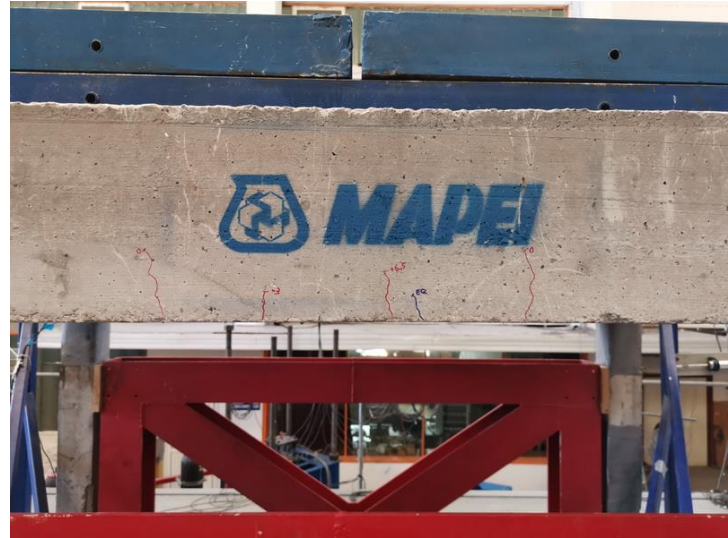
Fig. 12 – Cracking pattern in the longitudinal beam
