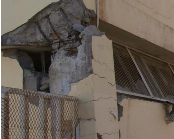
Fig. 1 – Collapsed short-column during the 2003 earthquake in Algeria [19]
