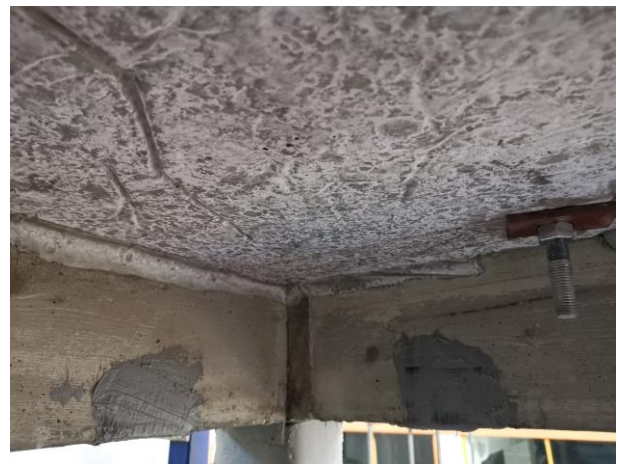
c. Collar for the anchorage (inside view)
