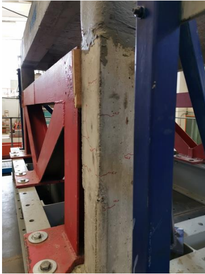
Fig. 11 – Damage in the columns
