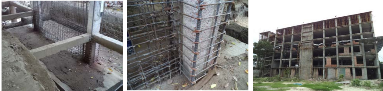
a) New RC shear wall and strengthening of shallow foundation, b) Column jacketing, c) Structural work
