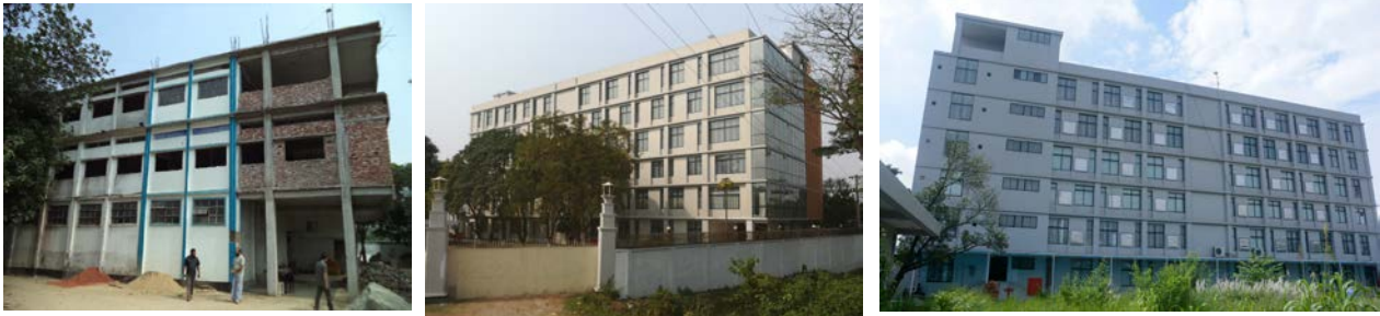
Fig. 1 - Existed building (left) and the building after retrofit (center and right) Source: JICA project
