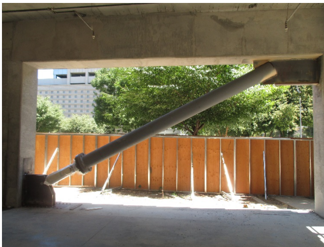
Fig. 19 –Seismic retrofitting using viscous dampers
