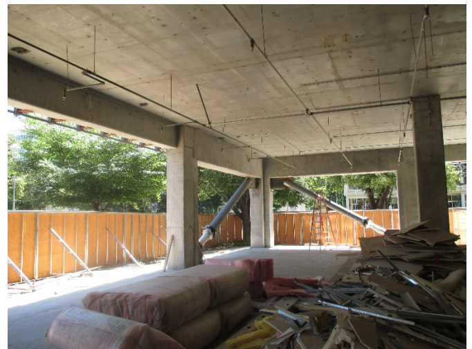
Fig. 19 –Seismic retrofitting using viscous dampers
