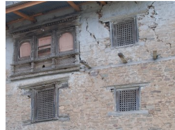
(d) Diagonal cracks propagating from the corners of openings
