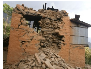
(b) Delamination caused due to separation of two layers of walls followed by out of plane failure.
