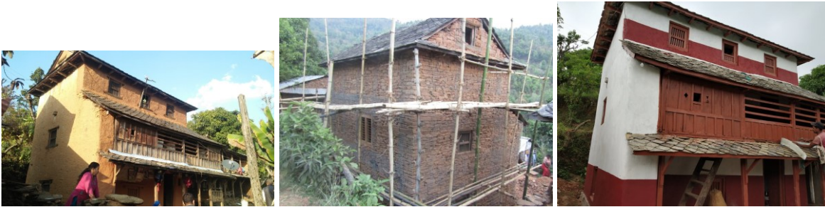
Fig. 5 – A building before (left), during (middle) and after (right) retrofitting (© NSET, 2015)
