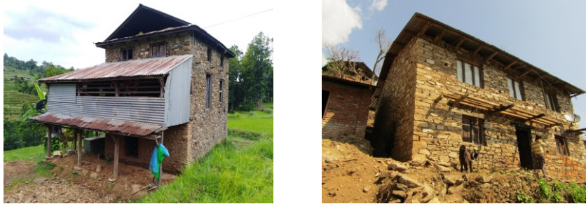
Fig. 1 - Typical stone masonry houses in mud mortar in rural Nepal. (©NSET)
