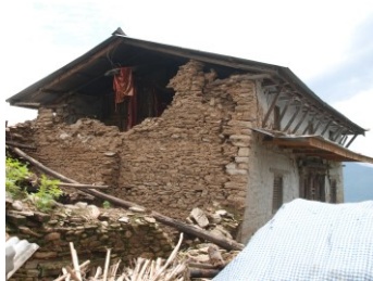
(c) Failure of masonry gable walls and separation of corners
