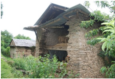
(a) Out of plane failure of orthogonal and gable walls.
