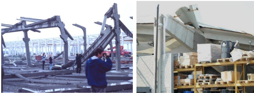
Figure 1: Damaged precast RC frames
