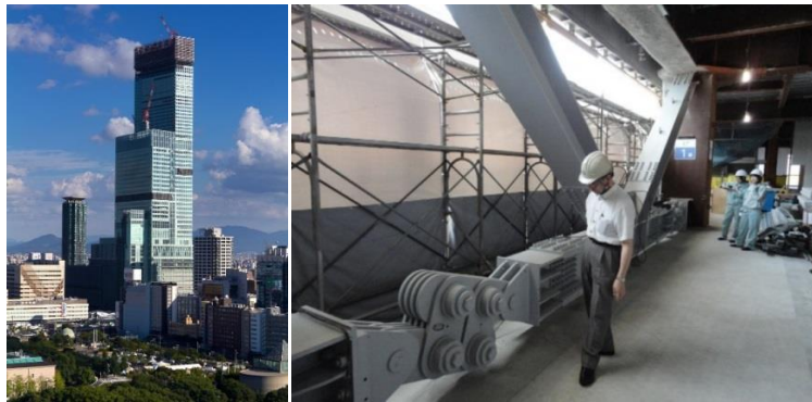
Figure 4. Japan tallest building Harukas 300, with Rotation Friction Dampers
