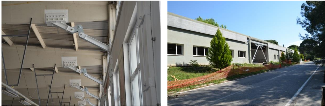
Figure 16. Photos of retrofitted structure
