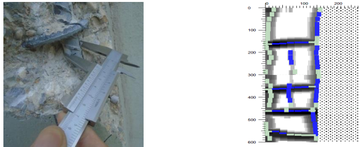
Figure 7. Identification of column reinforcement with clearing the cover and ferro-scan.
