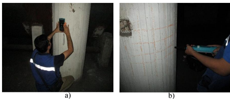
Fig. 2 – a) Rebar detection and b) Rebound hammer test on a concrete column
