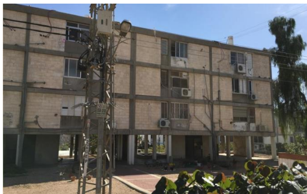
Fig. 1- “Train”-type building before retrofit
