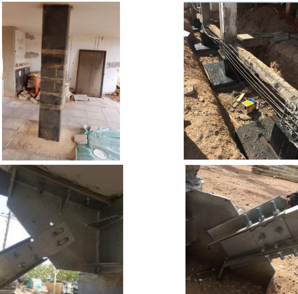
Fig. 11- Construction execution, clockwise from top left: RC column FRP jacketing, foundation retrofit, and steel brace details.
