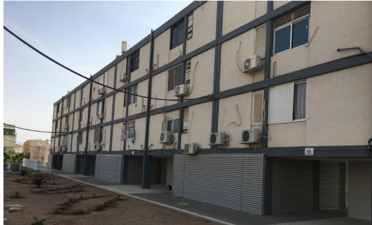
Fig. 12- Final appearance of structure after completion of retrofit
