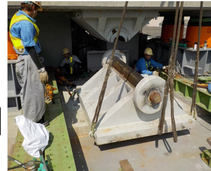
Fig.18 – Removal of existing steel bearing
