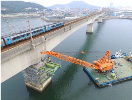
Fig.16 – Overview of retrofit
