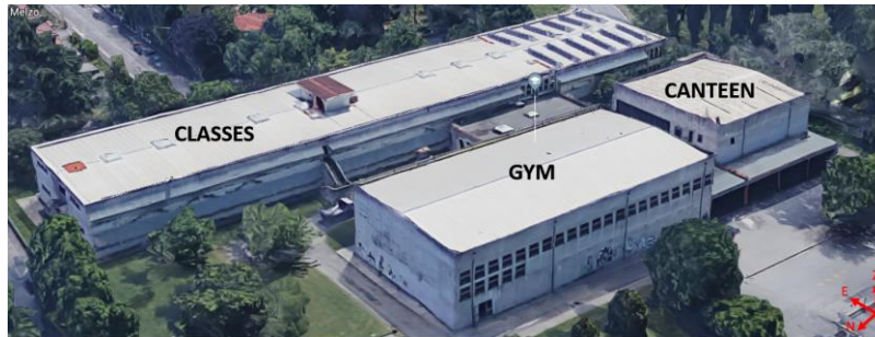
Fig. 1 – Structure overall view
