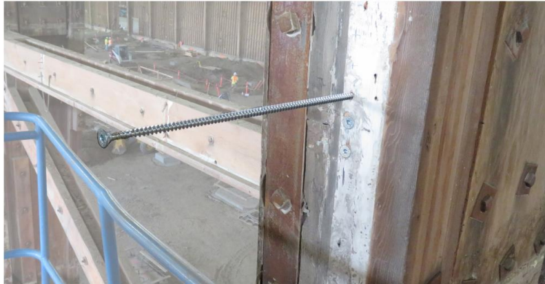
Fig. 10 - Fully threaded screw during installation
