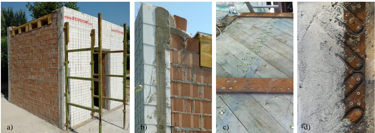
Fig.4 – a) One-story building specimen b) Detail of the retrofitting technology applied c) Timber floor d) Detail of the connection between the timber floor and the concrete layer
