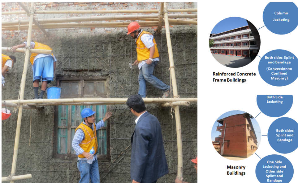
Fig.5 Retrofit option adopted to strengthen the vulnerable school buildings
