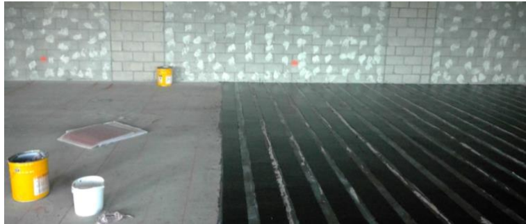
Fig. 2 – Unidirectional CFRP Placement
