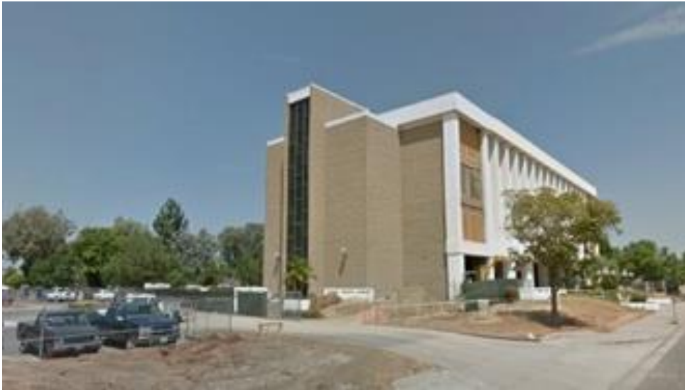
Fig. 3 – Case-Study Building during construction
