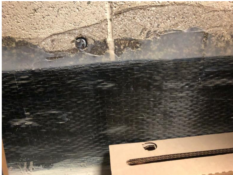
Fig. 4 – CFRP placement in the Case-Study Building
