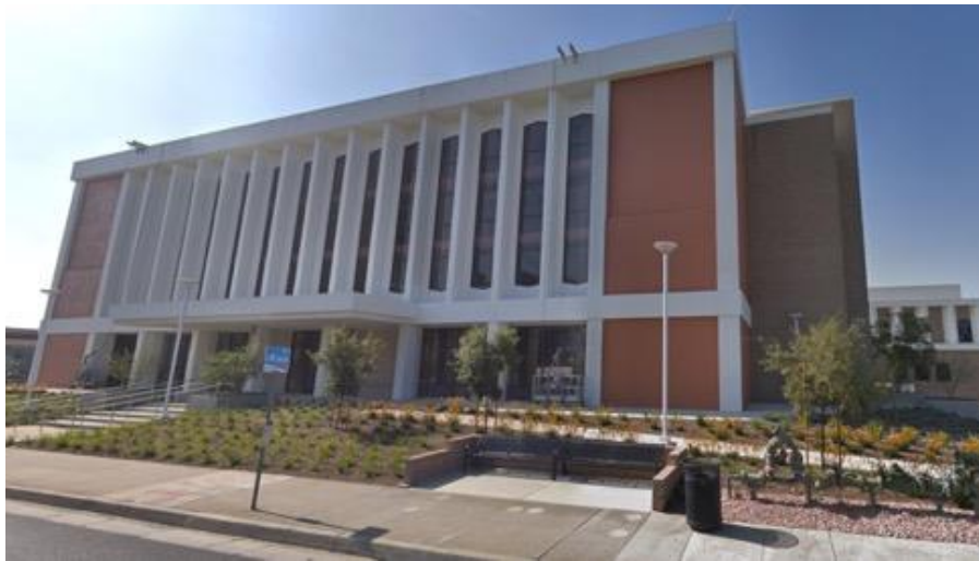
Fig. 1 – Present State of the Case-Study Building
