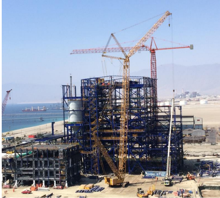
Fig. 2 – Photo of the Boiler Building during construction.
