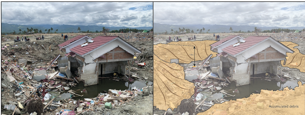
Fig. 3 – Deposited debris thickness in the accumulation zone of the Petobo Landslide.
