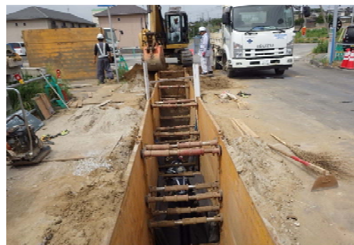
Fig. 28 – Excavation work in Hirai-tobu
