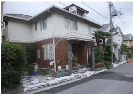
Fig. 1 - Settled and tilted houses in Urayasu City
