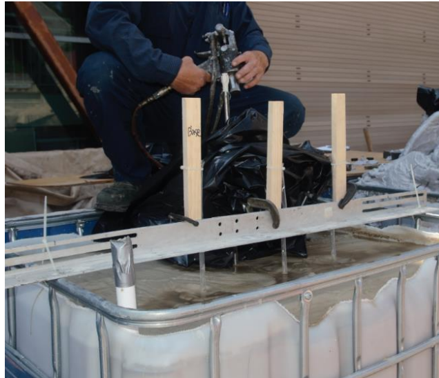
Fig. 3 – Polymer injection in each container
