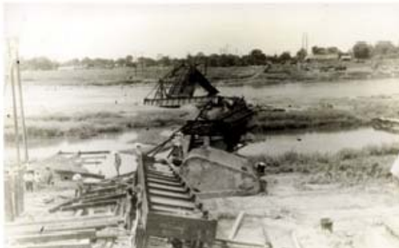
Fig.9 Rail way bridge fell down by liquefaction
