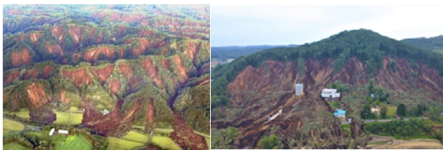
Fig.24 Collapses slopes and flowed earth
