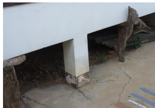
Fig.2 - Settlement of a shallow foundation
