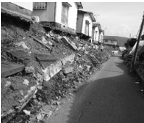
Photo 2 – An example of the collapsed retaining wall
