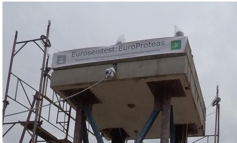
Fig. 4 –The one end of the wire rope and the load cell attached to the roof slab.
