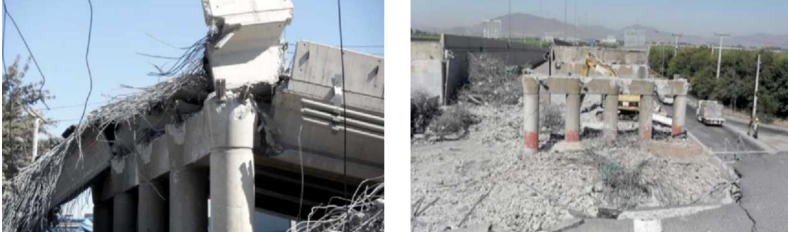
Fig. 8. Damage patterns in Overpass Lo Echevers and Miraflores.
