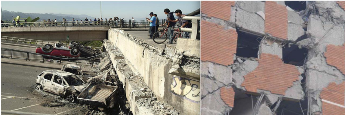
Fig. 10. Collapsed bridge in Concepcion shown on the left and damaged apartment building on the right.
