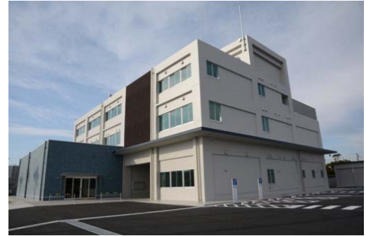
Fig.3 – The whole view of the facility
