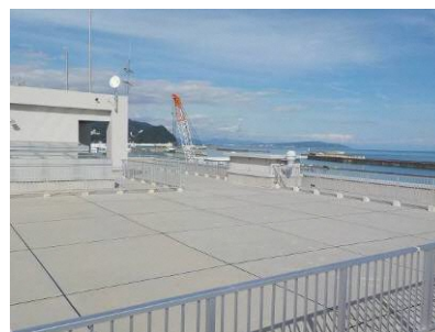
Fig.17 – Rooftop evacuation space
