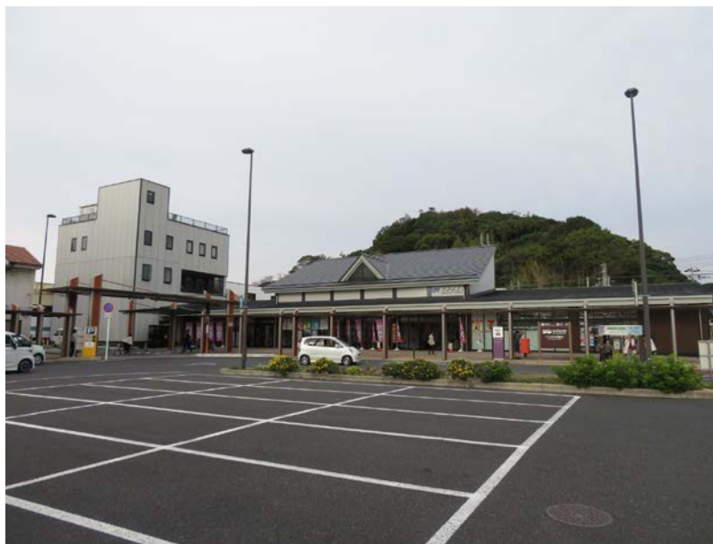
Fig.4 Photograph of exterior
