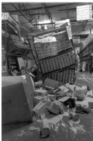
(a) Collapsed storage racks and fallen contents during an earthquake (FEMA, 2005)
