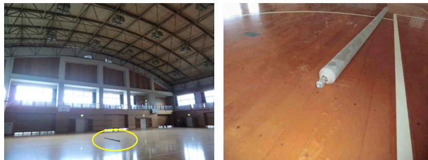
Fig.1 Damage of a High School Gymnasium after the Second Quake
