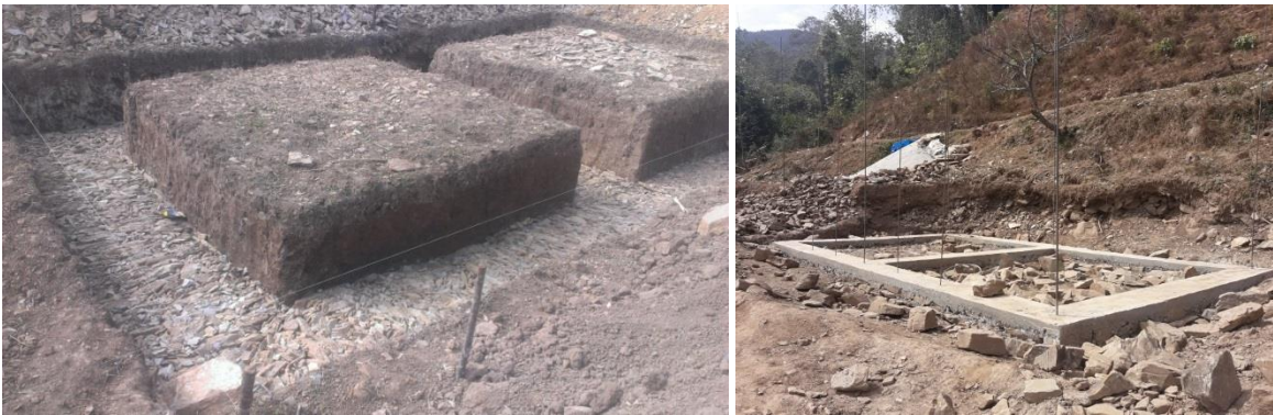
Figure 6. Excavation for foundations, left; construction up to plinth level, right.
