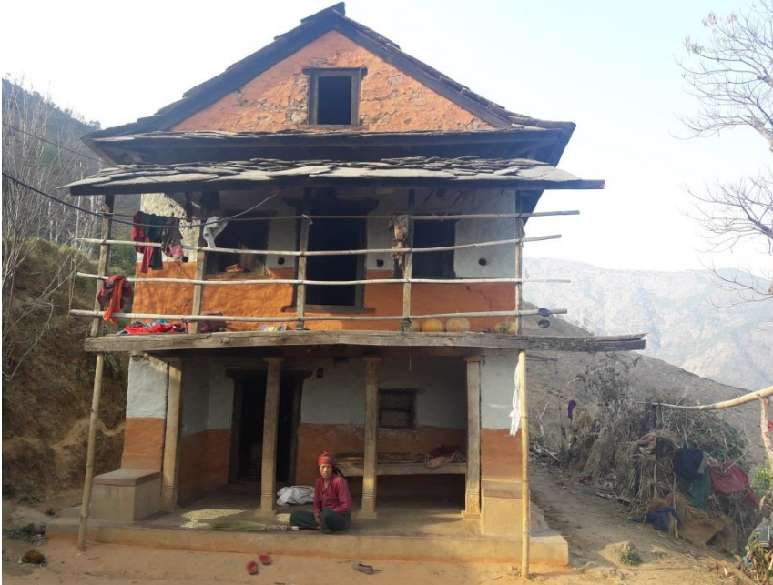
Figure 1. Typical single-family house found in Bijulikot prior to the earthquakes.
