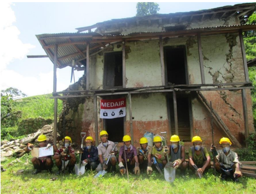
Figure 5. House ready for demolition.
