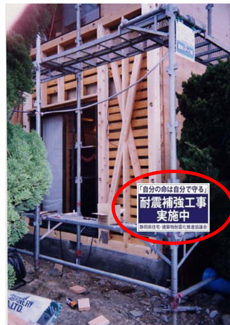
Fig.7— A signboards describing “Protect your own life Under seismic retrofit construction”
