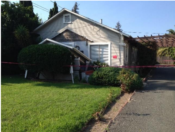
Fig. 2– One-story single-family crawlspace house that came off of its foundation in the 2014 South Napa earthquake. The gas meter was damaged and the toppled porch roof blocked the front door creating an unsafe condition. (Photo credit: CEA)
