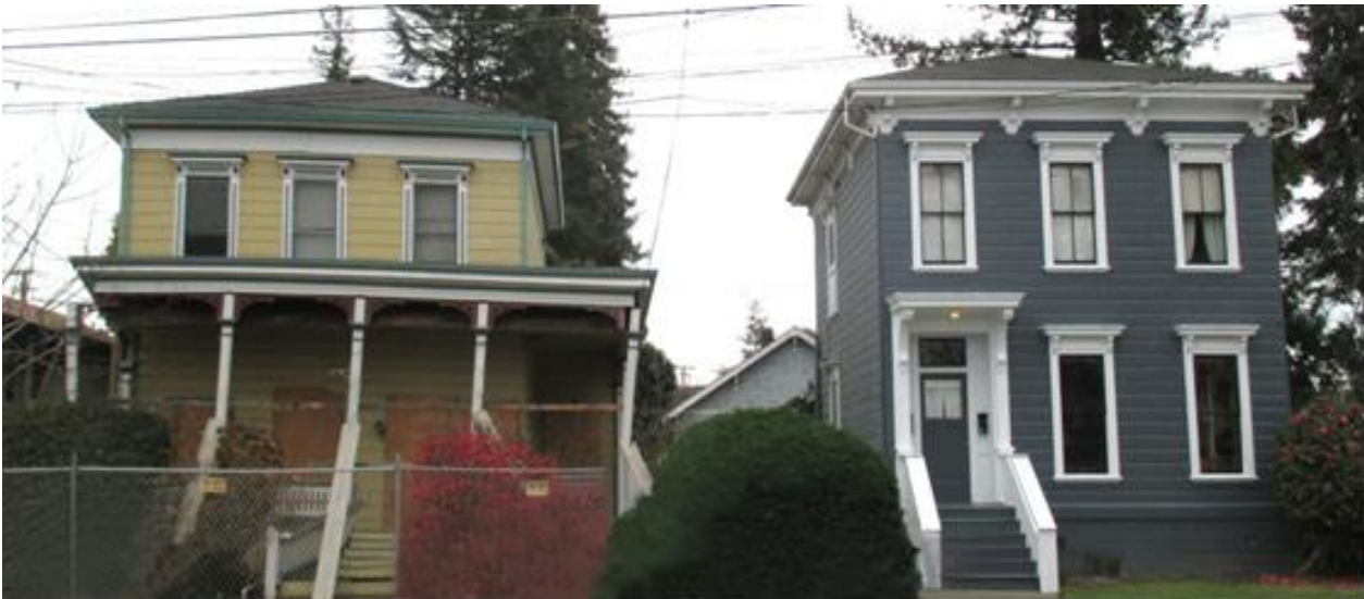
Fig. 1– The un-retrofitted house on the left came off its foundation during the 2014 South Napa earthquake (California, United States) rendering the house uninhabitable for over two years. The retrofitted house on the right had damage but the occupants were able to stay in their house during repairs. (photo credit: CEA).
