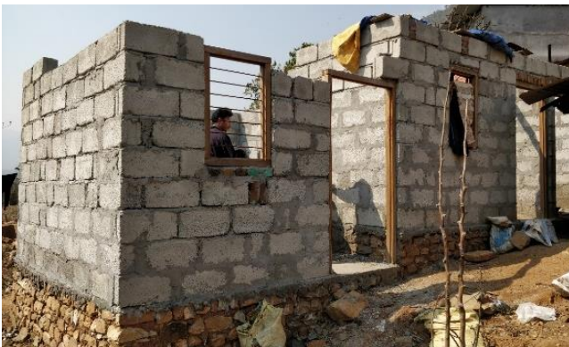
HCB house construction in Pokhara
