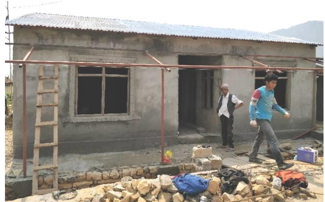
Steel frame structure with hollow concrete blocks infill walls in Parbat
