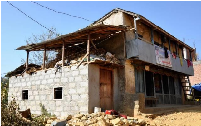
HCB extension to a stone masonry house in Dhading
