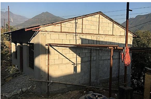
HCB house with steel truss for roof in Nuwakot
