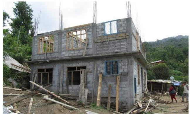
RC frame building with HCB infill in Dolakha
